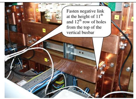
Install double positive link between positive vertical busbars in Slave No.2 C32442.002 and Slave No.3 C32442.003 using 8x M10X35 screws, washers and nuts as shown on the picture.
