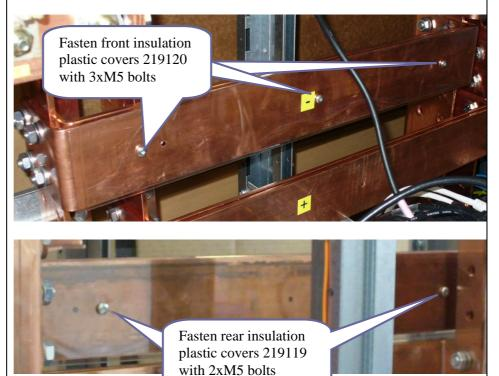
Install double negative link with plastic covers between negative vertical busbars in Master C32442.001 and Slave No.1 C32442.002 using 8x M10X35 screws, washers and nuts as shown in the picture.
