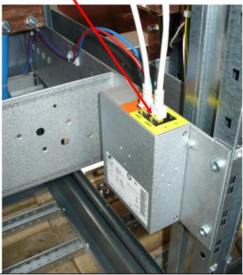
3.3 Remove End termination plugs from bottom CAN BUS connection in the PowerRack in Slave No.2 C32442.002 and from CAN BUS connection in Smartpack in Slave No.1 C32442.002
