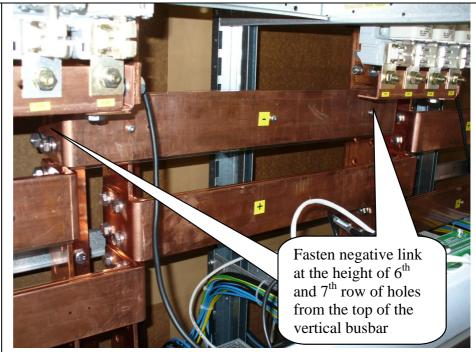
Install double positive link between positive vertical busbars in Slave No.1 C32442.002 and Slave No.2 C32442.002 using 8x M10X35 screws, washers and nuts as shown on the picture.
