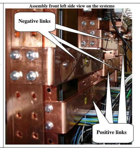
1.4 As the system is positively grounded negative distribution links need insulation to prevent shortcut between them and cabinets.
